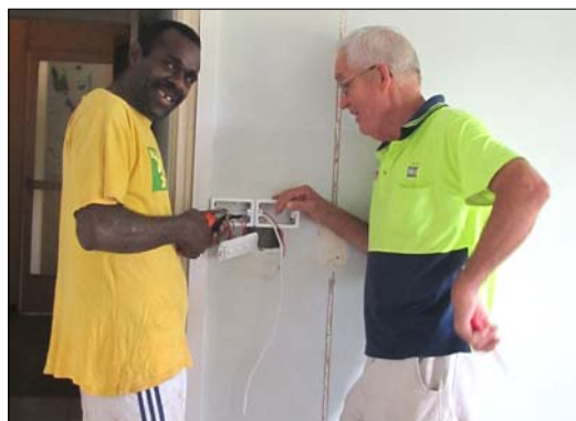
Lewi and Peter installing new switches
