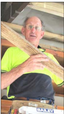
Gerry de Vos installing a new ceiling in Hilltop
