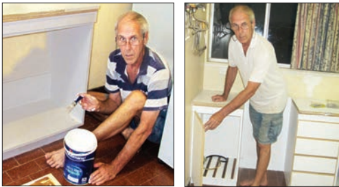
Peter painting cupboards and installing doors
